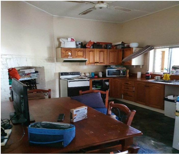
Kitchen. Rear wall and sink etc to be removed.
