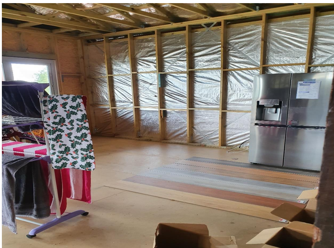
Extension added to rear, this part to be the new kitchen.
