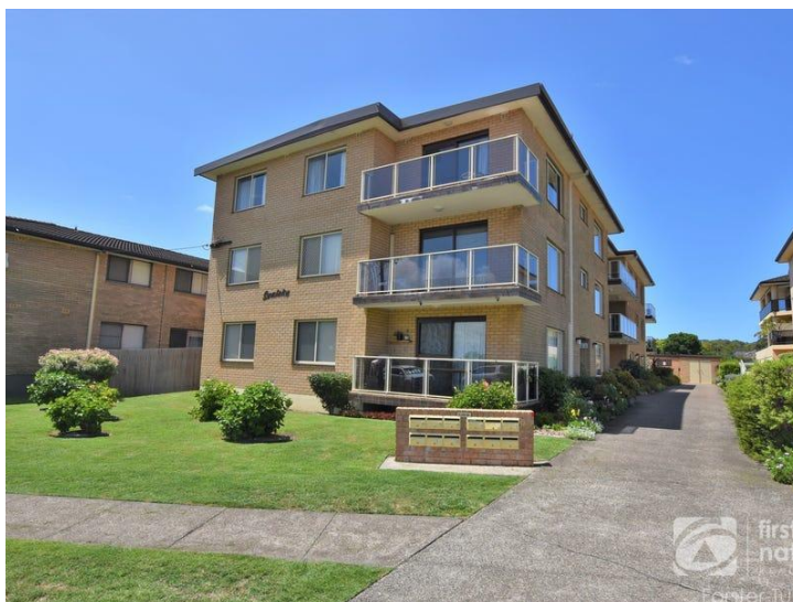
View of the Apartments Building at 82 Little Street, Forster.
