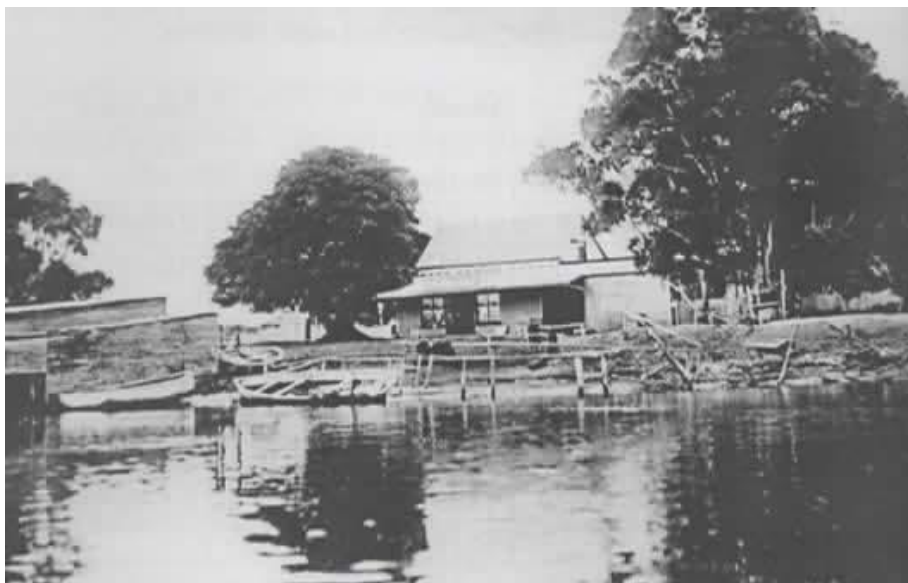
R.R. Breckenridge's store in Little Street, Forster
